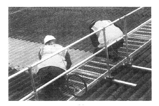
Workmen wearing harnesses attached to a work positioning line which is fitted to the staging
